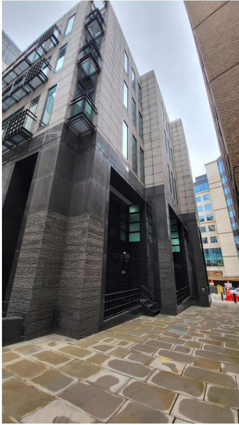
Image 6: The southern elevation of the southern block within Ashentree Court.
